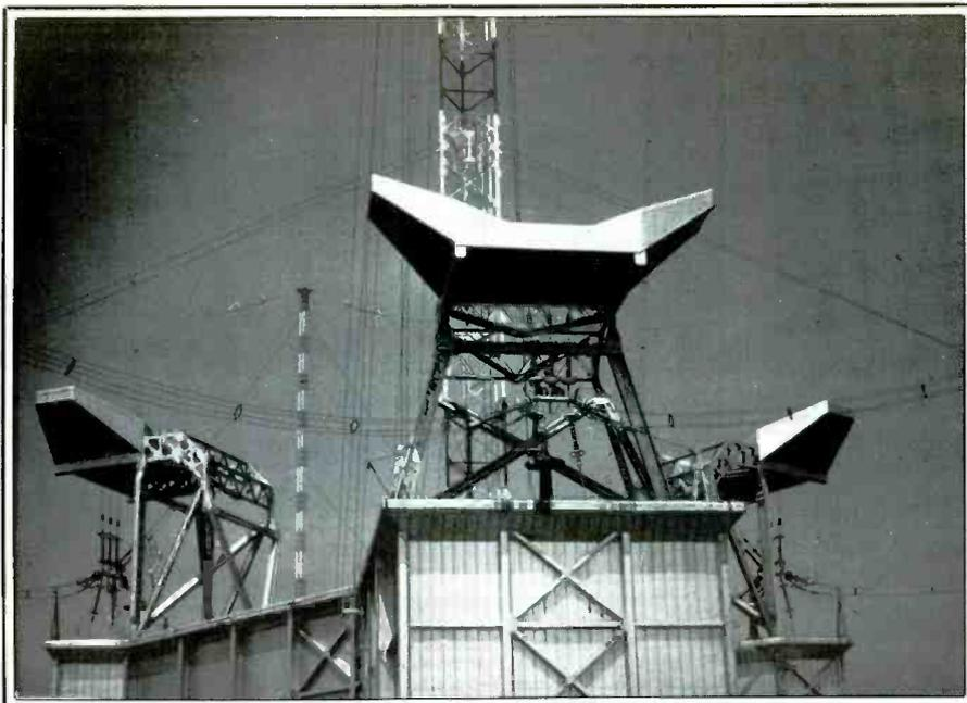
Ice guards are required throughout the system. These protect the helix houses from being damaged by icing.
