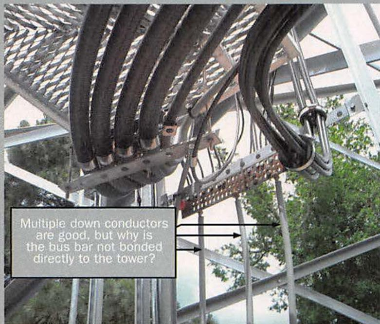
Multiple down conductors are good, but why is the bus bar not bonded directly to the tower?
