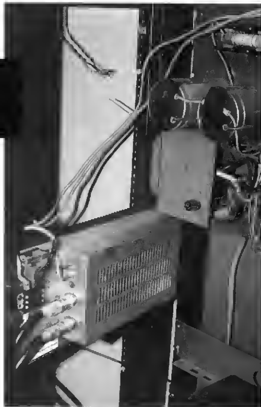
The W1KKF repeater transmitter generates about 30 W, which is boosted to 100 W, thanks to this amplifier.
