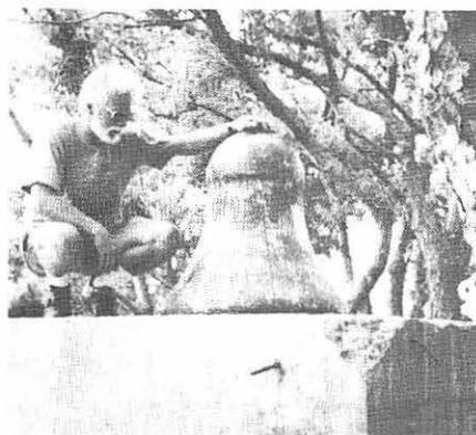
Blackman examining the base of Fessenden's tower. The swivel enabled the tower to move with the wind, keeping the weather strains from snapping the guy wires.
