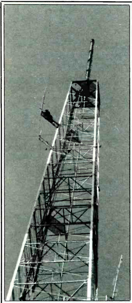
Installing an Army MARS receiving antenna 375 feet up; WDLI-TV transmitter tower located in Canton, Ohio. (Photo by John S. Papay, K8YSE/AAR5WI)
