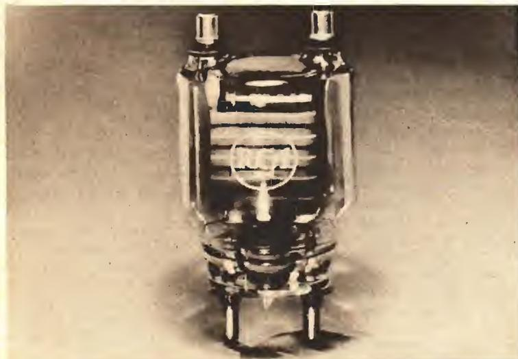
Amateurs are advised that it is now practical to operate the RCA-833-A at a full kilowatt input in plate-modulated class C telephony service, without the use of forced-air cooling. Typical data for this new natural-air-cooled operation are yours for the asking. Write to Commercial Engineering, RCA, Harrison, N. J.
