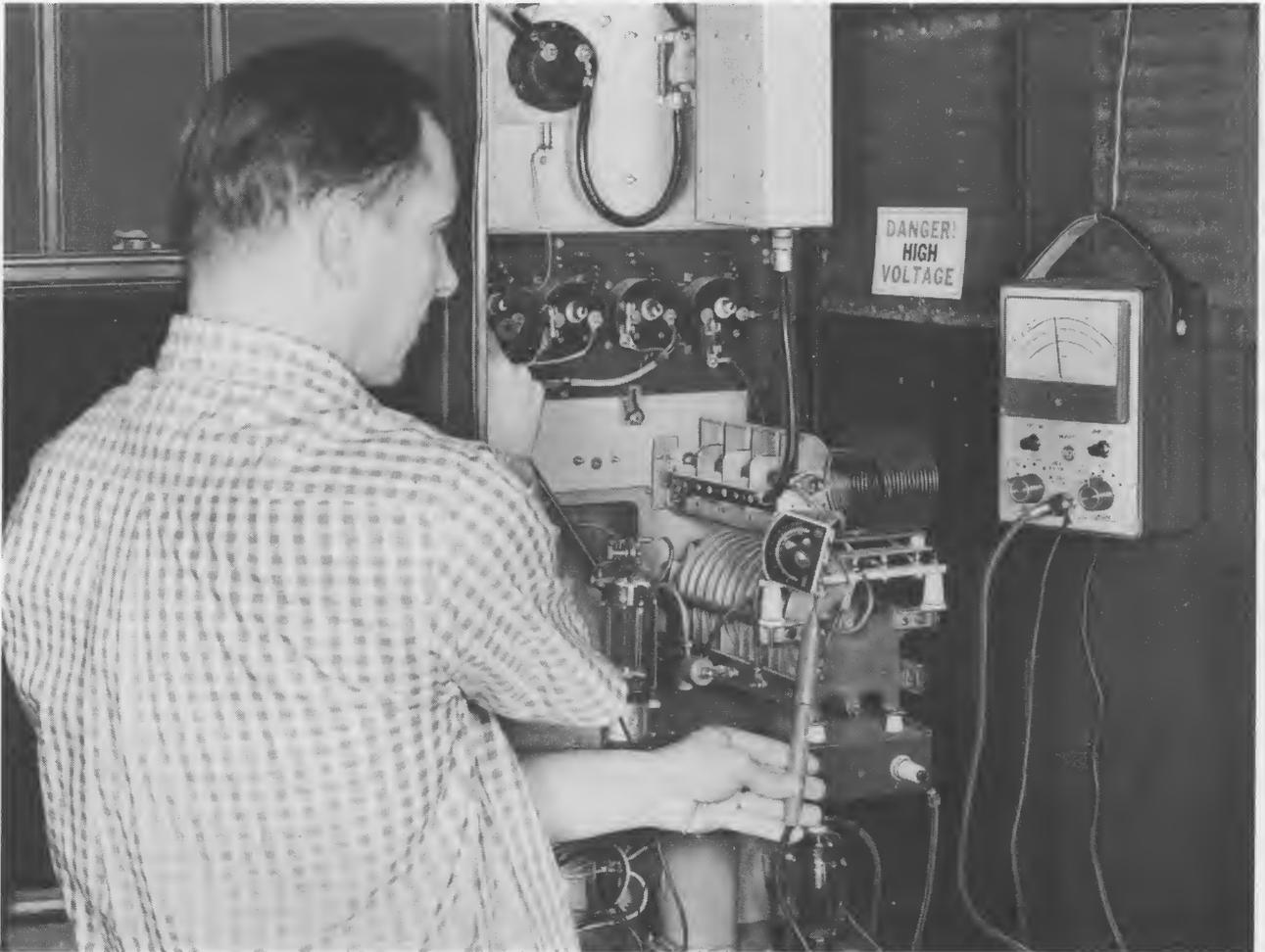
When connected to a wavemeter circuit, the VoltOhmyst makes an excellent rf-tuning indicator. Here, W2IYG uses the WV-77C and WG-301A Crystal-Diode Probe during neutralizing of final amplifier.
